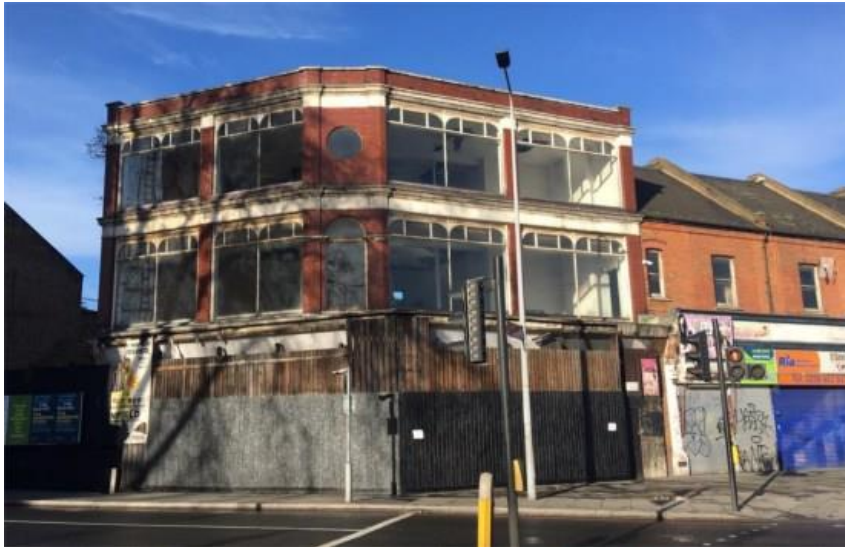
PICTURE 1: The vacant three-storey Corner building
